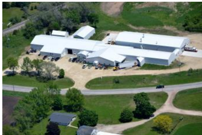
Darley's Ohler Plant in Janesville, IA
